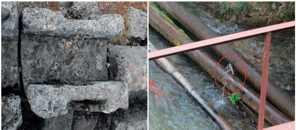
Fig. 15. Ancient sluice gate - Modern water tap (photo author).
