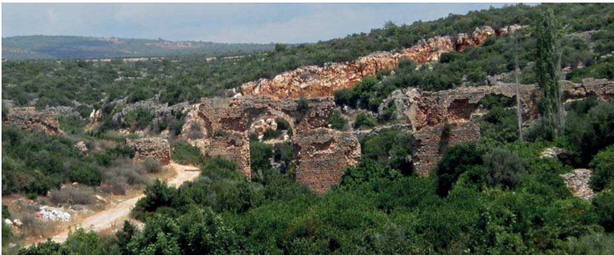
Fig. 8. Yemişkumu B aqueduct bridge (photo author).
