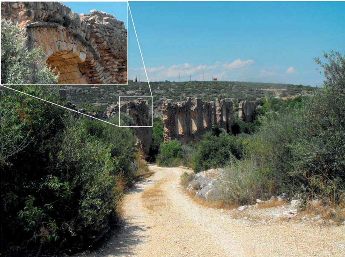
Fig. 5. Tirtar aqueduct bridge (photo author).
