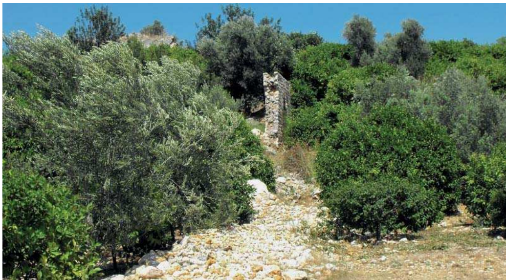
Fig. 13b. Kuru Dere B aqueduct bridge (photo author).
