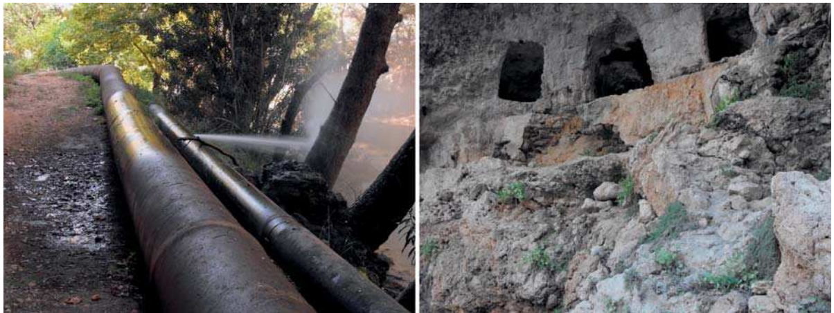
Fig. 14. Modern pipeline below ancient channel (photo author).
