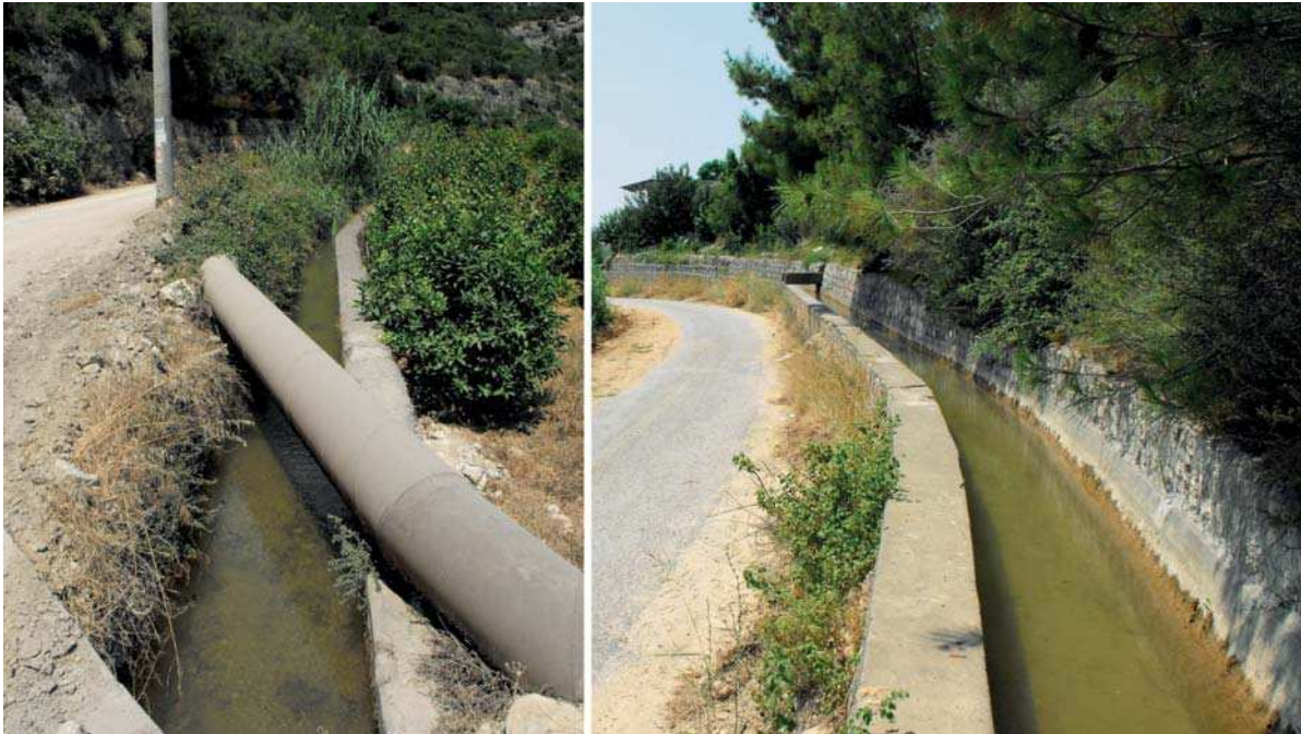
Fig. 3a. Modern pipeline (photo Author). Fig. 3b. Concrete channel (photo author).
