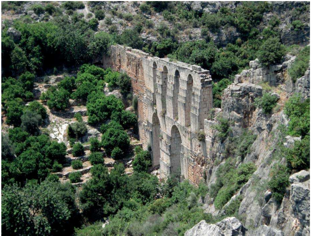
Fig. 4. Limonlu aqueduct bridge (photo author).
