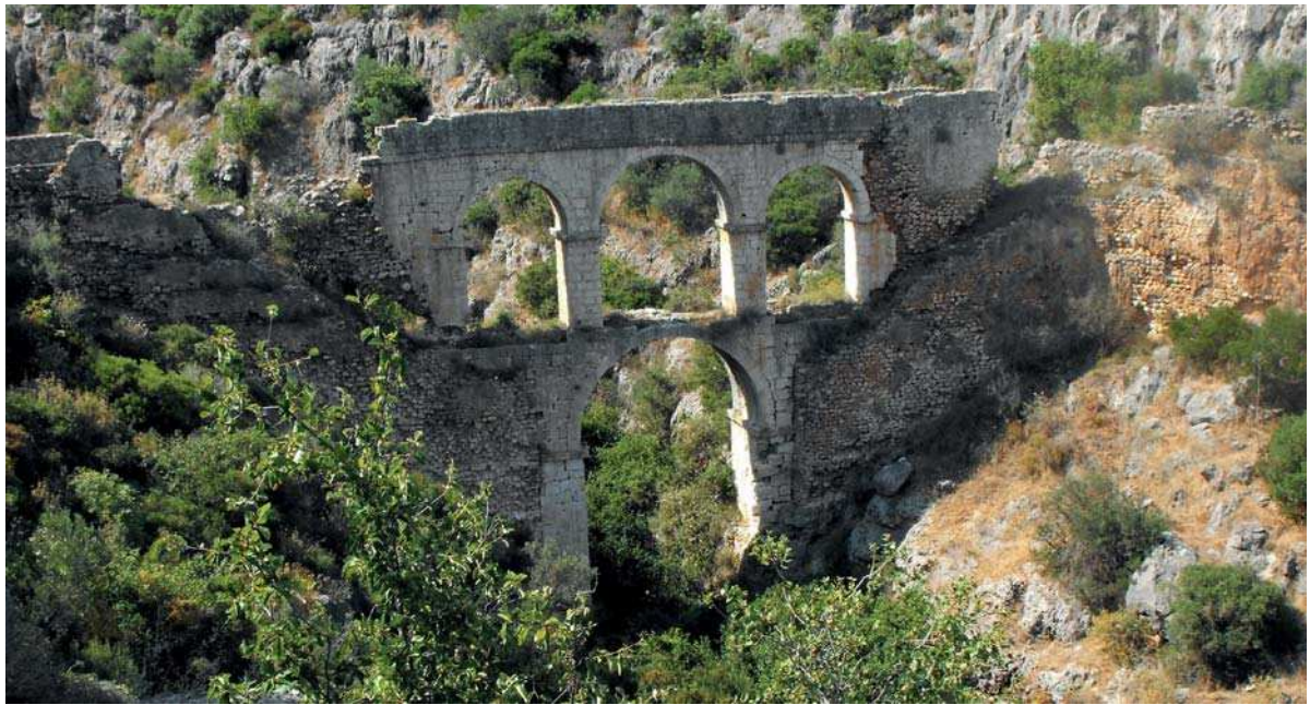
Fig. 6. Kumkuyu aqueduct bridge (photo author).
