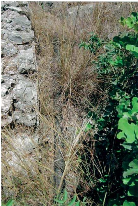
Fig. 10. Modern pipeline in channel specus (photo author).
