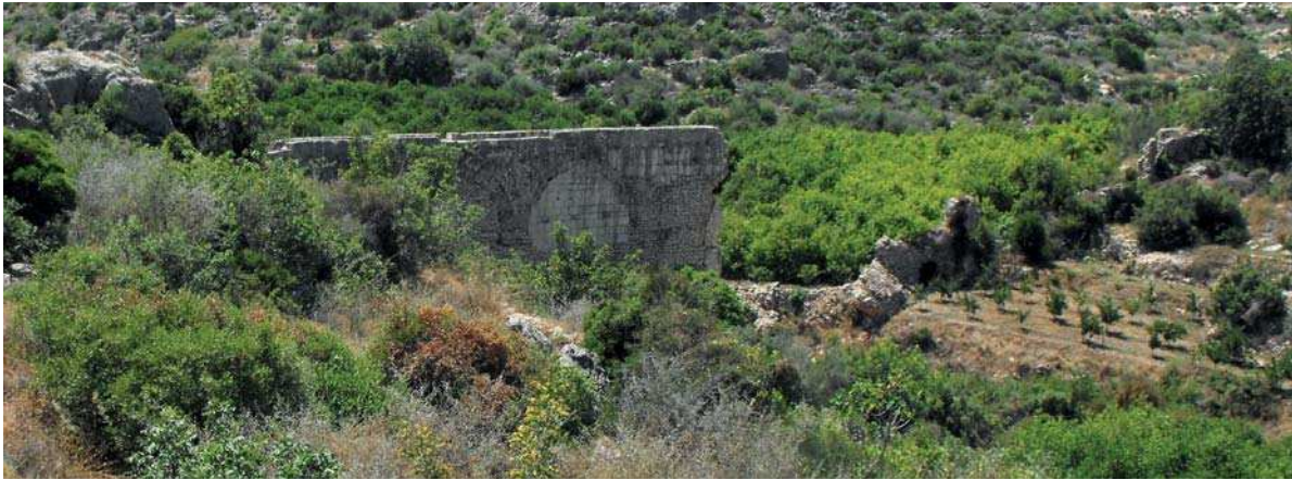
Fig. 11. Yemişkumu D aqueduct bridge (photo author).
