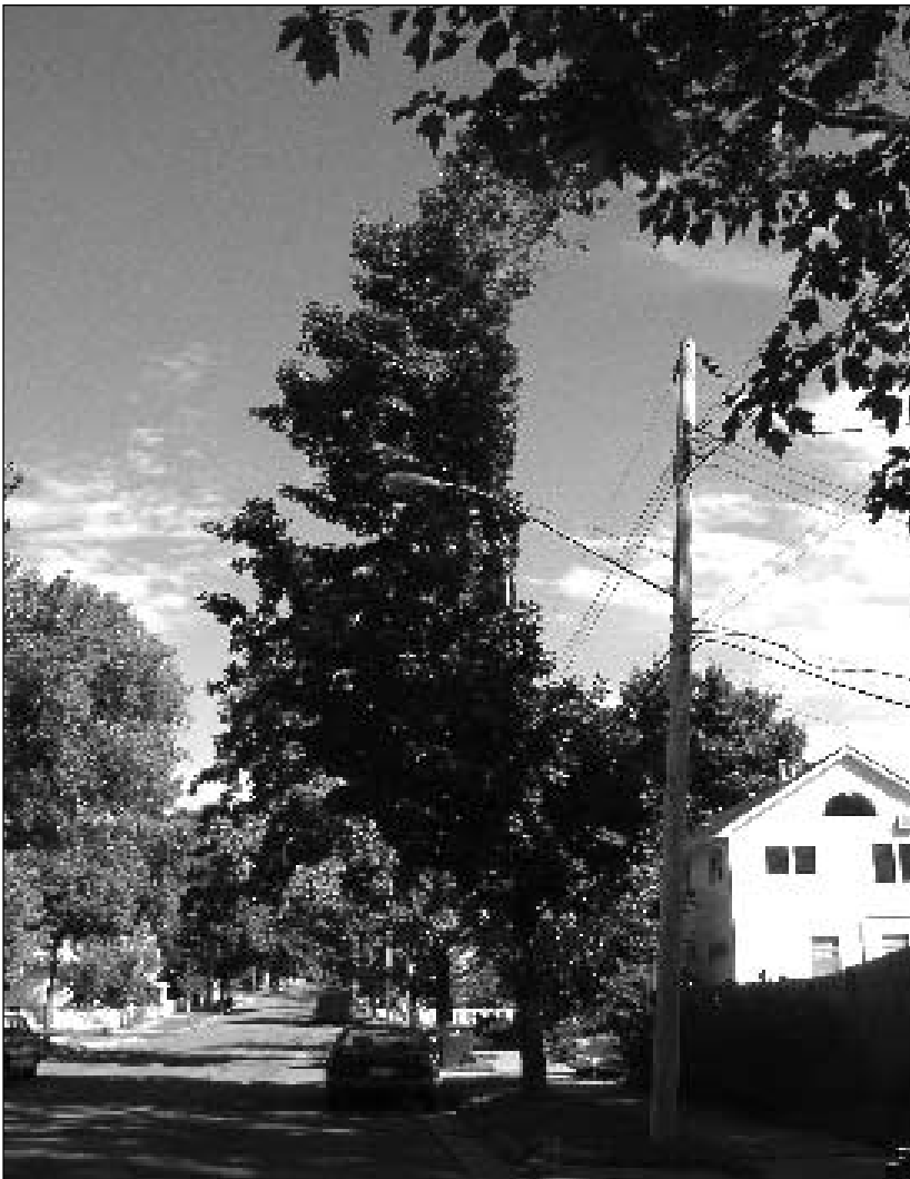
Figure 12—Large trees planted under power lines can require extensive pruning, which increases tree care costs and reduces the benefits of those trees, including their appearance.
