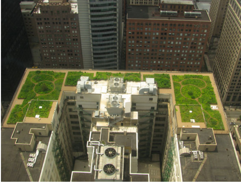
Fig. 4.4 Chicago city hall green roof (TonyTheTiger, http://commons.wikimedia.org/wiki/Main_Page )
