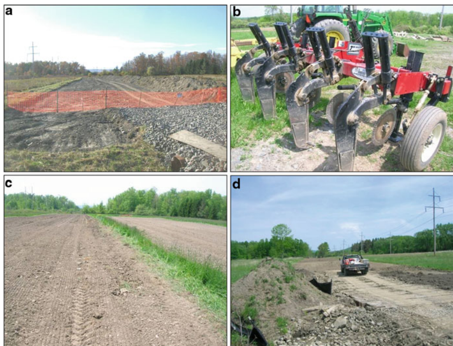
Fig. 12.3 Representative photos after pipe installation from pipeline project right of way. Photo a Agricultural land after pipe burial. Fall, 2008. Topsoil stockpiled on right. Photo b Unverferth zone-till ripper used to decompact ROW in agricultural land areas. Photo c Agricultural land (see Photo a ) after to drilling of grass mix. Spring, 2009. Photo d Wooden timber mats across ROW protect wetland soils. Soil berms and silt curtains control erosion
