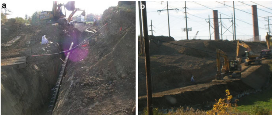
Fig. 12.1 Heavy machinery and soil disturbance during pipeline project right of way construction. Photo a Pipe installation in trench bottom across fallow land use type. Note vehicle traffic directly on top of subsoil spoil. Photo b Stripped topsoil segregated upslope from pipe in agricultural land use area. Vehicles shown backfilling subsoil spoil before topsoil
