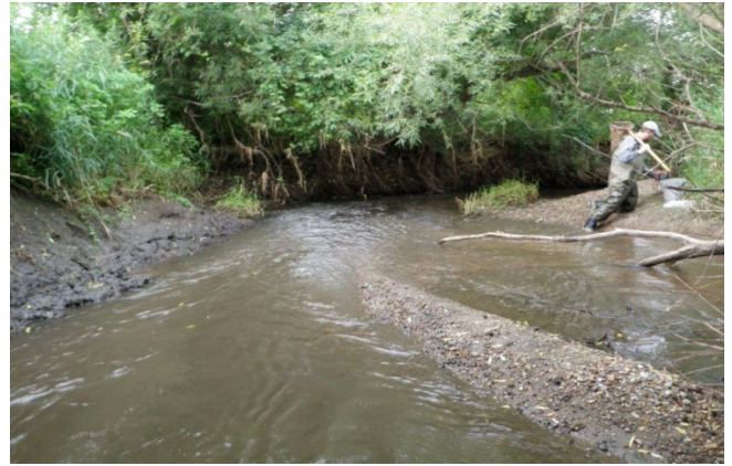
Image 6: Evidence of channel instability as bank erosion and mid-channel bars at 11LM008 on unnamed creek.
