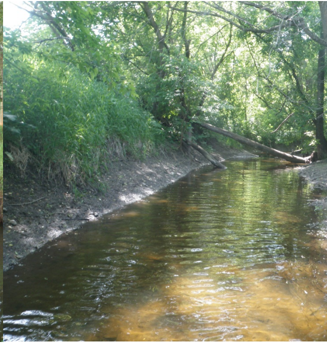
Image 12: Incised banks and shallow run filled with silt on Knowles Creek (June 13, 2011).
