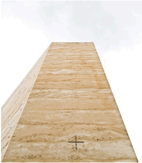
Fig. 5. Detail of layered local concrete facade.
