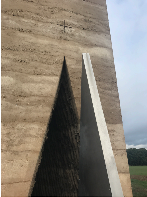
Fig. 4. Steel triangle door, ribbed texture interior, and layered concrete facade.
