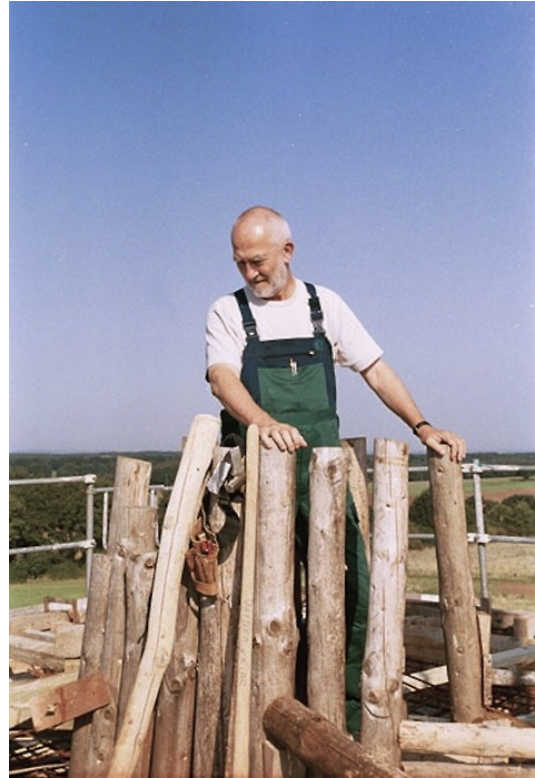
Fig. 8. Peter Zumthor building wigwam structure on site.
