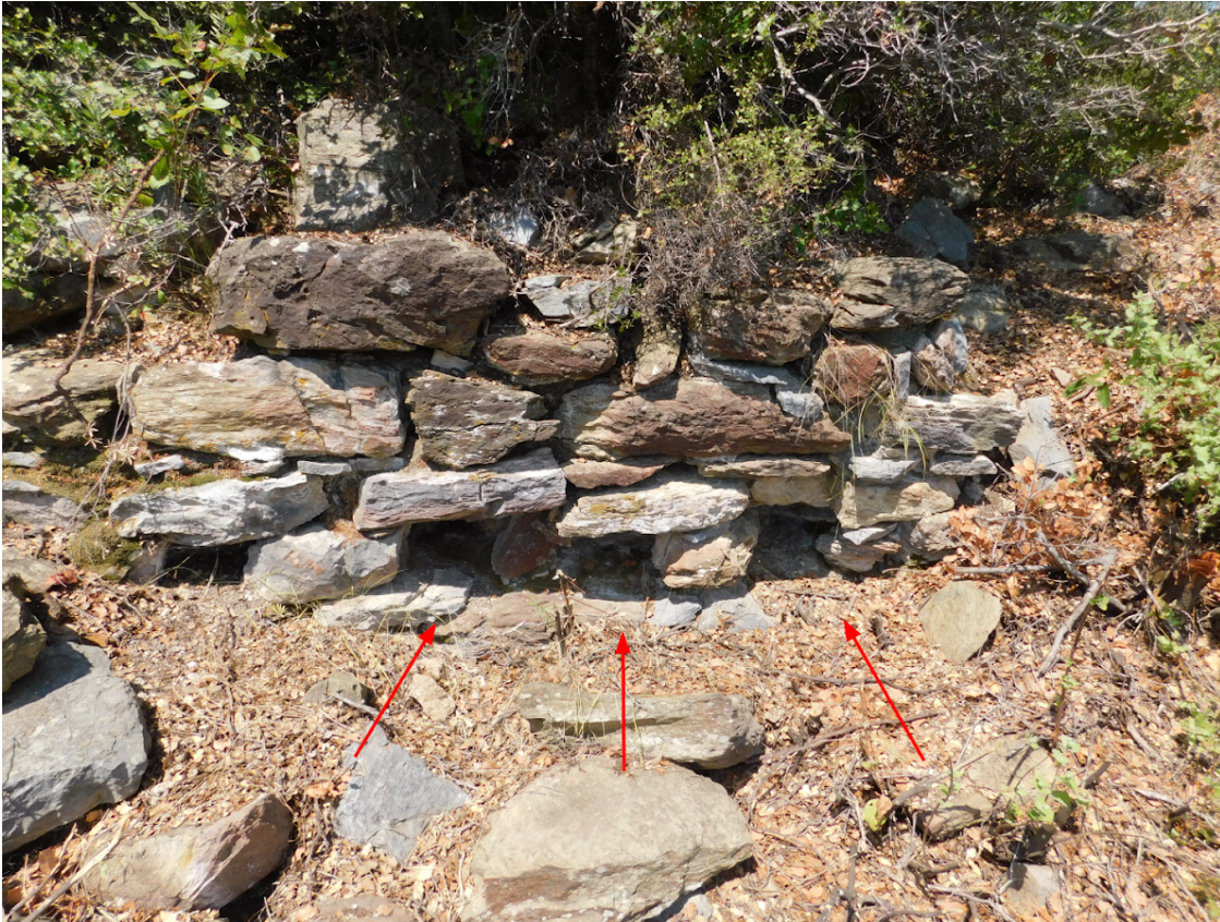
Figure 1. Wall with Beam Holes
