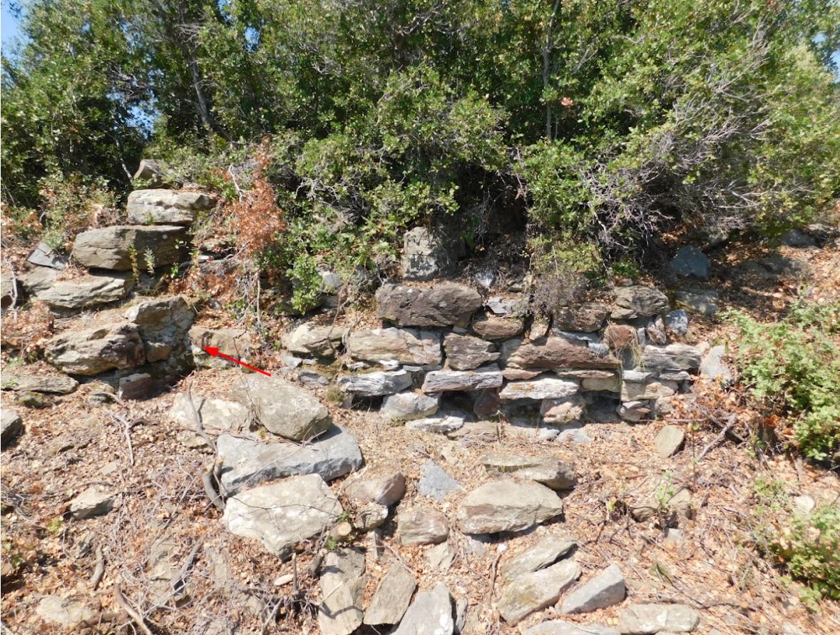
Figure 2. Wall and Southwest Corner
