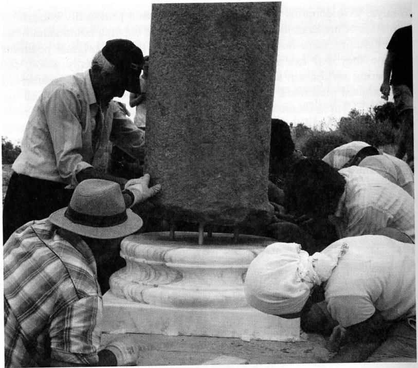
Figure 10-10. Colonnaded Street. Anastylosis of original column upon new base.
